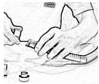
Assemble the ring & remaining parts of the connector to the conduit
