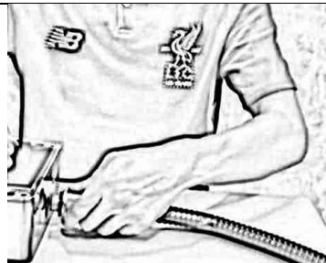
Open the opening in enclosure & insert the connector with the conduit
