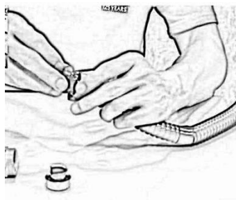
Assemble the sleeve into the conduit
