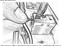
Unscrew the terminal screw in anticlockwise direction
