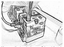
Unscrew the terminal screw & insert the wire in it & tighten in clockwise direction with a torque of 0.8Nm.
